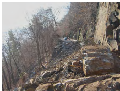
Figure 10. Photograph of the December 17, 2005, rockslide damage on the Alpine Approach Road in Alpine. Photograph courtesy of “Palisades Interstate Park - NJ Section.”
