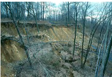
Figure 14. Landslide which destroyed Bellwood Farm Road, Bethlehem Township, Hunterdon County in 1989. Photograph by S. Stanford, N. J. Geological Survey.
