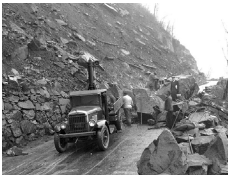
Figure 7. Photograph of a rockfall on Henry Hudson Drive March 8, 1933, in Bergen County. Photograph courtesy of “Palisades Interstate Park - NJ Section.”
